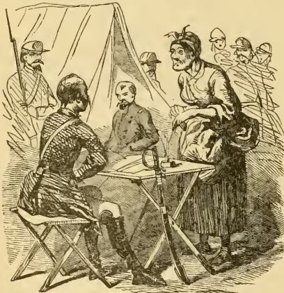
Settling a Claim
